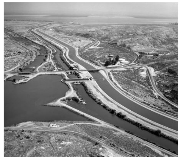
Record-breaking '83 Kern River flows successfully diverted into the California Aqueduct via the Kern River Intertie to avoid flood damage
