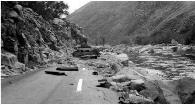
Flooding damage from the 1951 flood to Highway 178, which closely follows the Kern River down to Bakersfield
